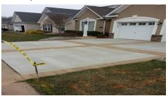
New driveway will include the removal of existing blacktop Meet existing pavers where applicable 4" stone sub-base, if needed and tamped 5" thick concrete driveway at 4000 psi with wire mesh ½" expansion joints along garage floor and sidewalk Saw cut control joints
